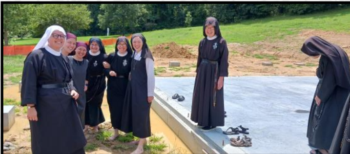
Trenches for plumbing
